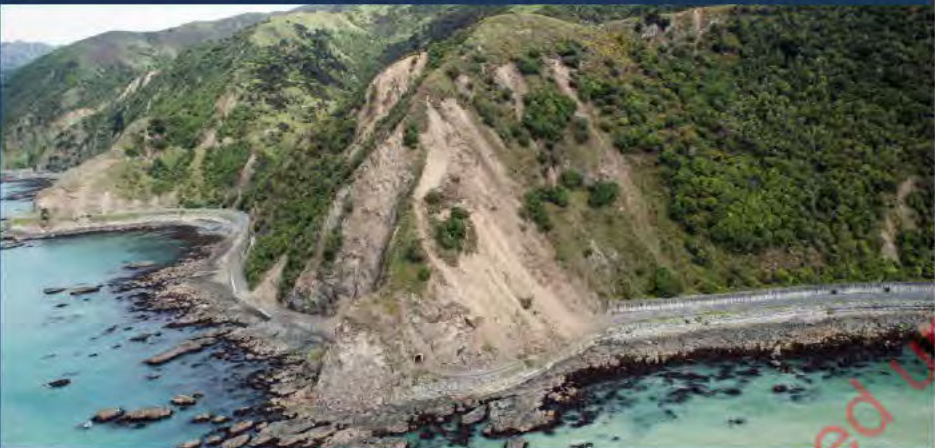
SH1 following 2016 Kaikōura EQ
