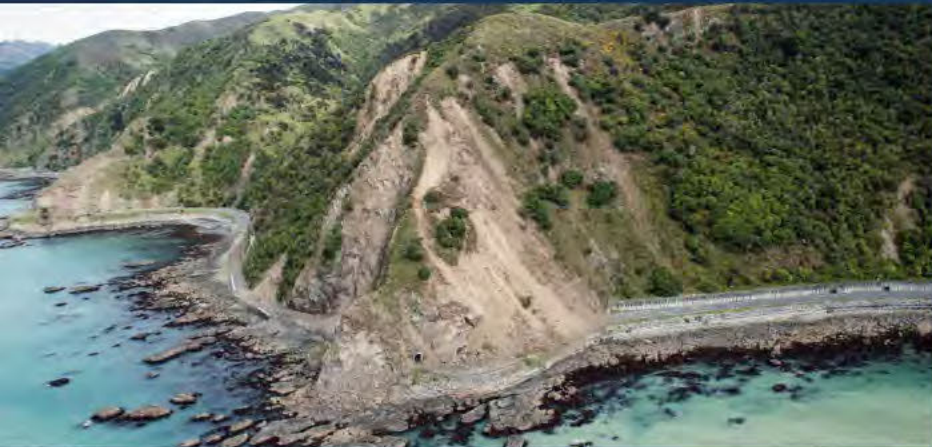
SH1 following 2016 Kaikōura EQ
