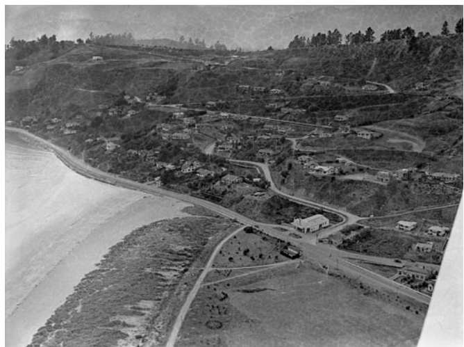
Figure 1: Tāhunanui Slump, Nelson – 1939. Tāhuna Beach in foreground with Rocks Road heading to north
