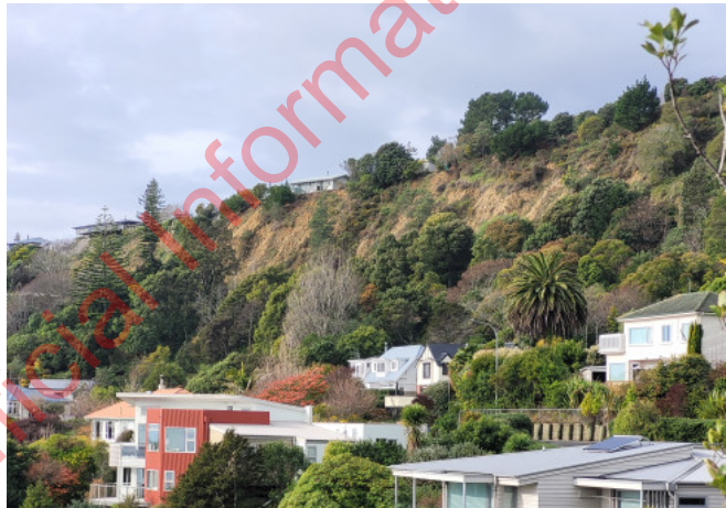
Figure 1: Tāhunanui Slump head scarp, Nelson 2023. Visible when flying into/from the northern approach
