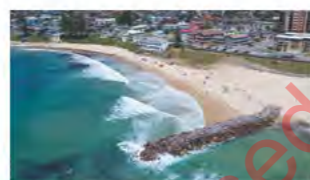
The new groyne at the Entrance Beach completed in December 2017.
