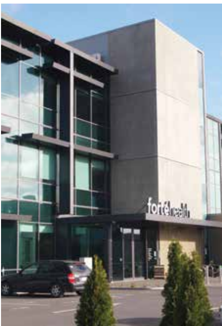
The Forté Health building was the first post-quake project to achieve a Green Star rating.
