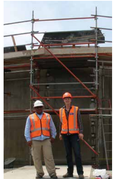
Farrukh Gondal, McConnell Dowell Project Engineer, and Andrew Stewart, SCIRT Civil Engineer, at Victoria Park's new reservoir on Cashmere, last month
