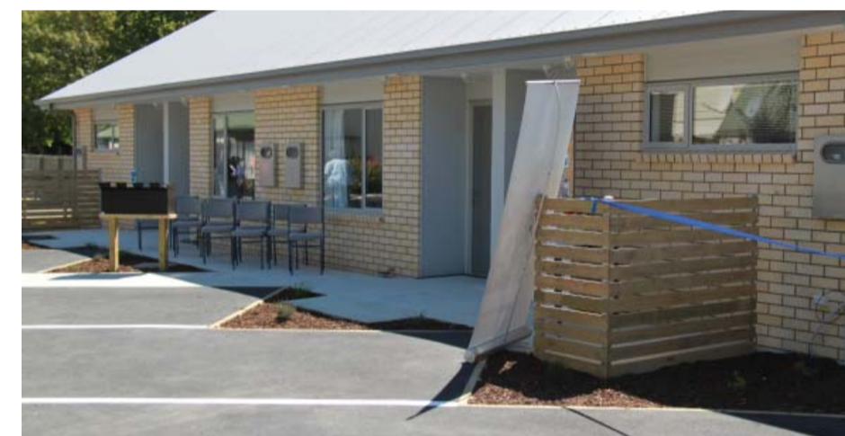
The new units at Harman Courts are warm, energy-efficient and ready to cater to the changing needs of tenants over their lifetimes.
