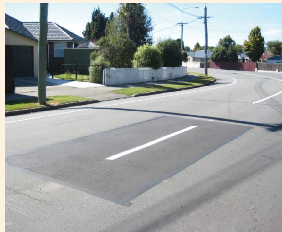
A patch repair on Ilam Road.
