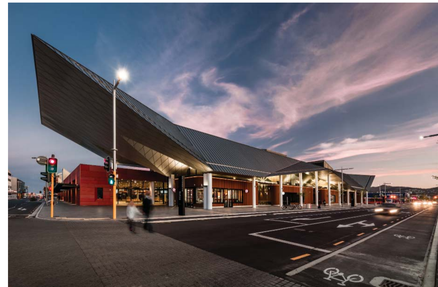
Stage One of the Bus Interchange opened in May 2015 with 8 of the 16 bus bays operational. Stage Two opened in October.
