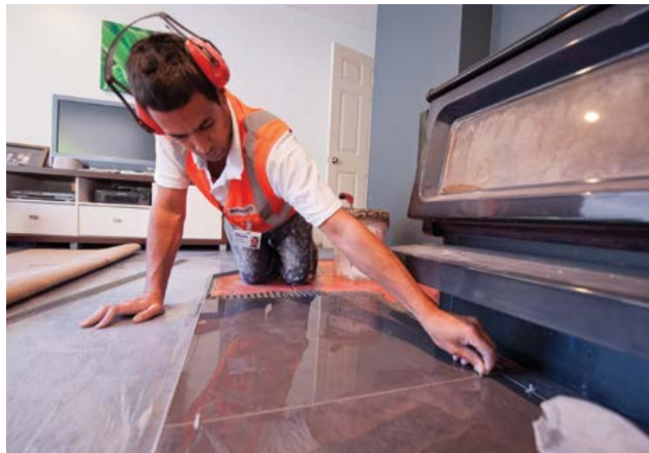
Re-tiling a fireplace surround as part of a CHRP repair.
