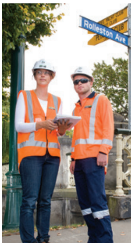
SCIRT McConnell Dowell crew members check plans for work at Armagh Street bridge.
