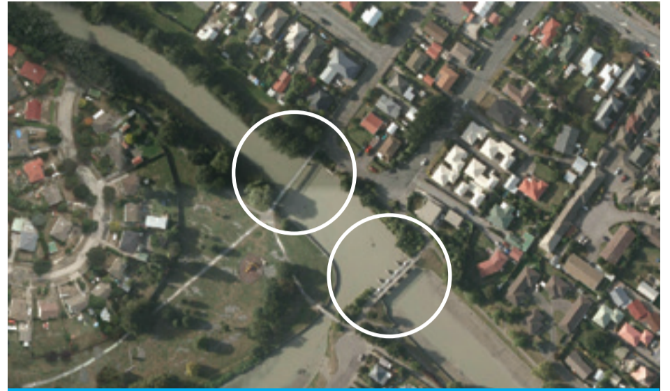
Aerial map showing the location of the Catherine Street footbridge (left) and the Woolston Tidal Barrage structure (right).
