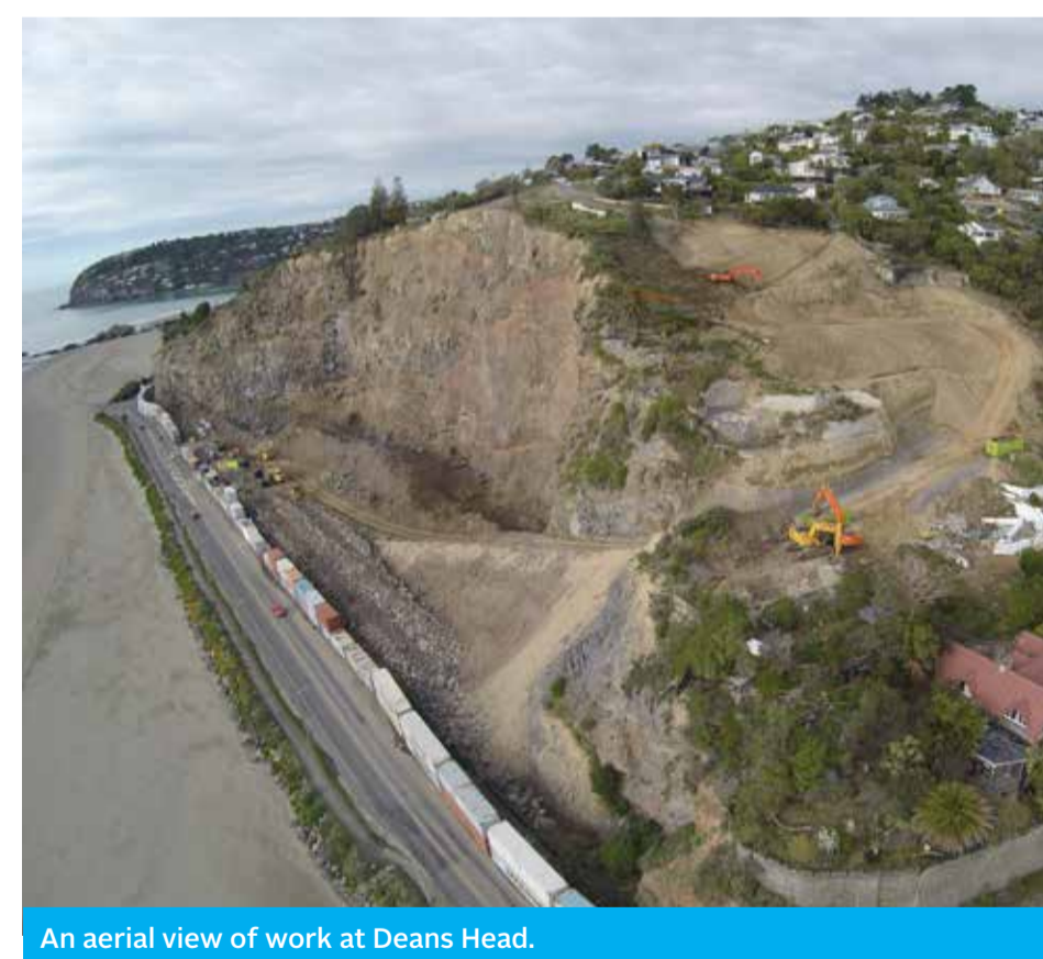
An aerial view of work at Deans Head.
