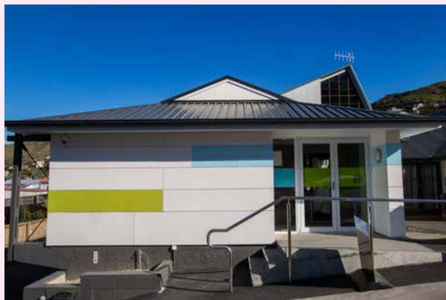
The new Lyttelton boardroom is available for community use.
