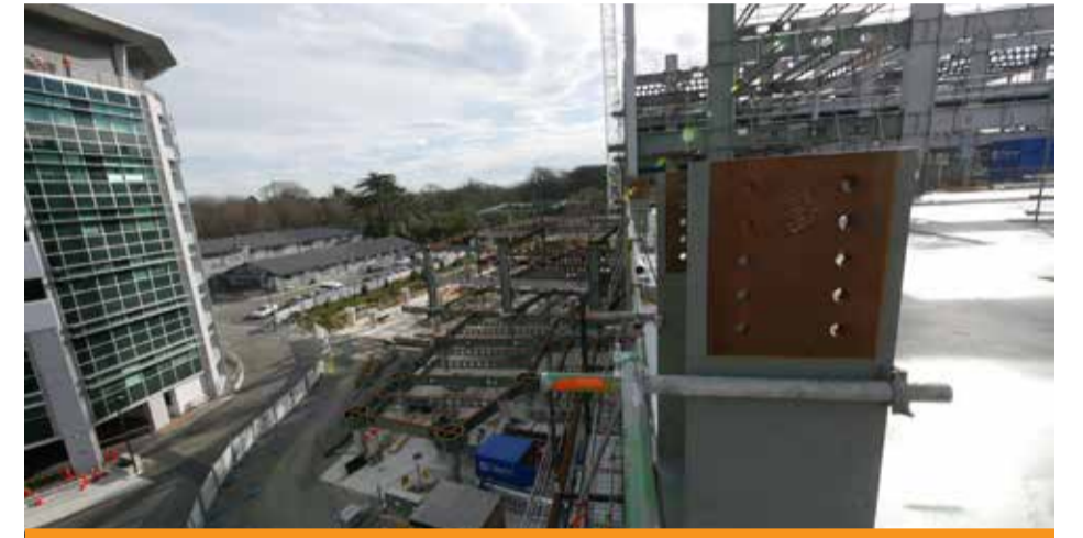
The record-breaking concrete foundation slab for the Acute Services building contains over 15,000 cubic metres of concrete, and enough reinforcing steel to stretch from Christchurch to Melbourne.
