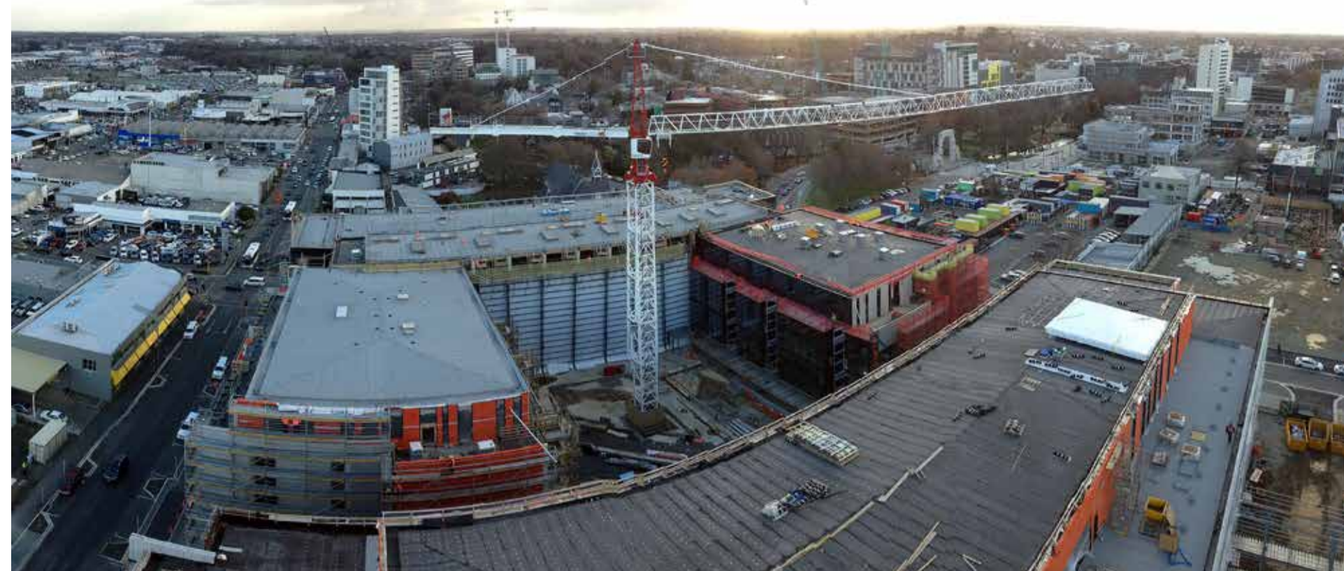
This staggering 'crane's eye view' shows the sheer size of the Emergency Services Building (foreground) and the three components of the Justice Building as it takes shape.
