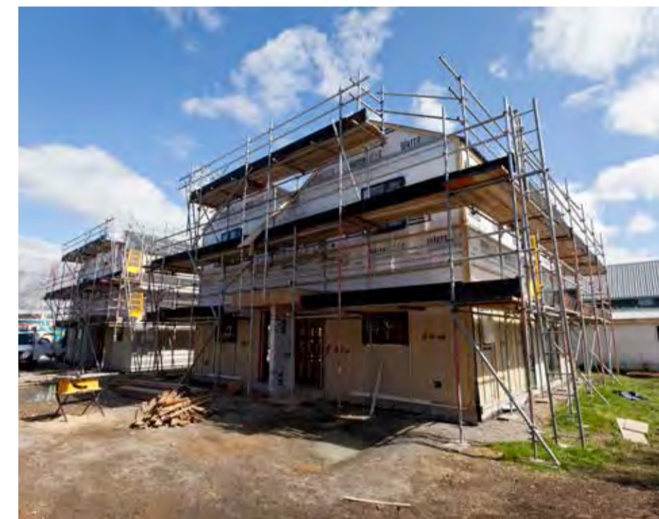
Housing New Zealand, which has completed its successful Canterbury Earthquake Recovery Programme, will continue to build new social housing right across Christchurch.
