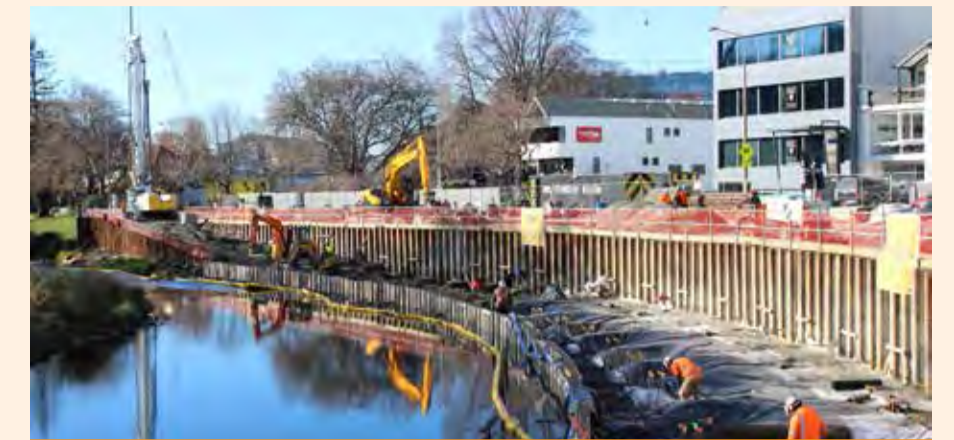
Work in progress: Piling is complete on the Earthquake Memorial and work has started on the reinforced concrete beams that will tie the piles into the main structure.
