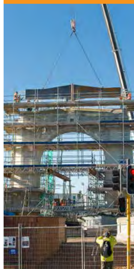
SCIRT workers lowering an 8.2-tonne beam into the Memorial Arch on the Bridge of Remembrance.
