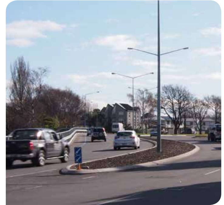
Fitzgerald Avenue after repair
