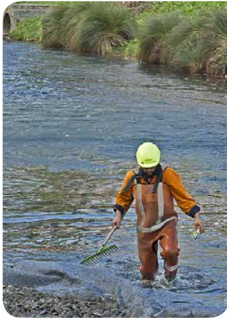
Avon River works, image courtesy of City Care
