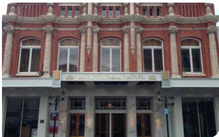
Isaac Theatre Royal façade
