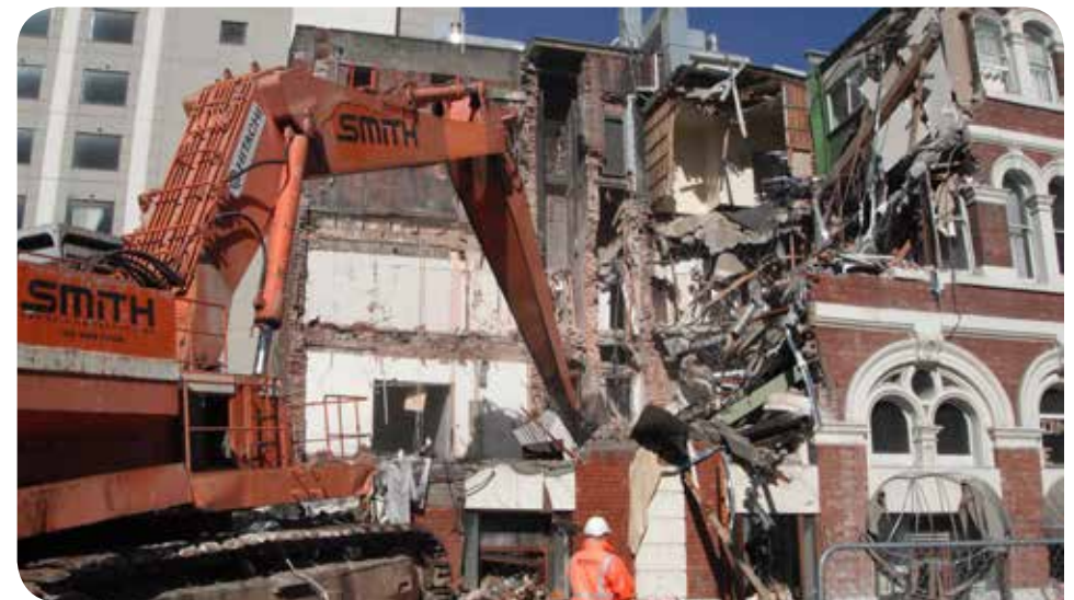
Demolition in progress
