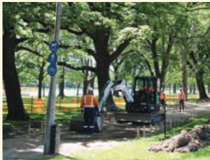
Council contractors widen the shared path parallel to Hagley Avenue from two to four metres. The work has been planned to minimise any impact on the trees.
