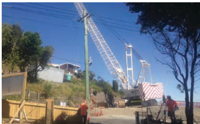
Top: Images from Unmanned Aerial Vehicles help identify potential hazards when planning difficult cliff-top demolitions. Bottom left: Cranes with long-reach booms provide a safer distance between the cliff edge and contractors. Bottom right: Aerial footage provides insight into the precarious nature of some cliff-top properties involved in CERA's property clearance programme.
