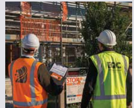
Fletcher EQR and EQC staff on site during home repair.
