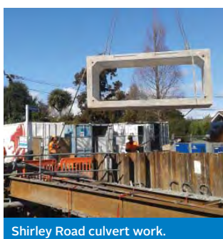
Shirley Road culvert work.
