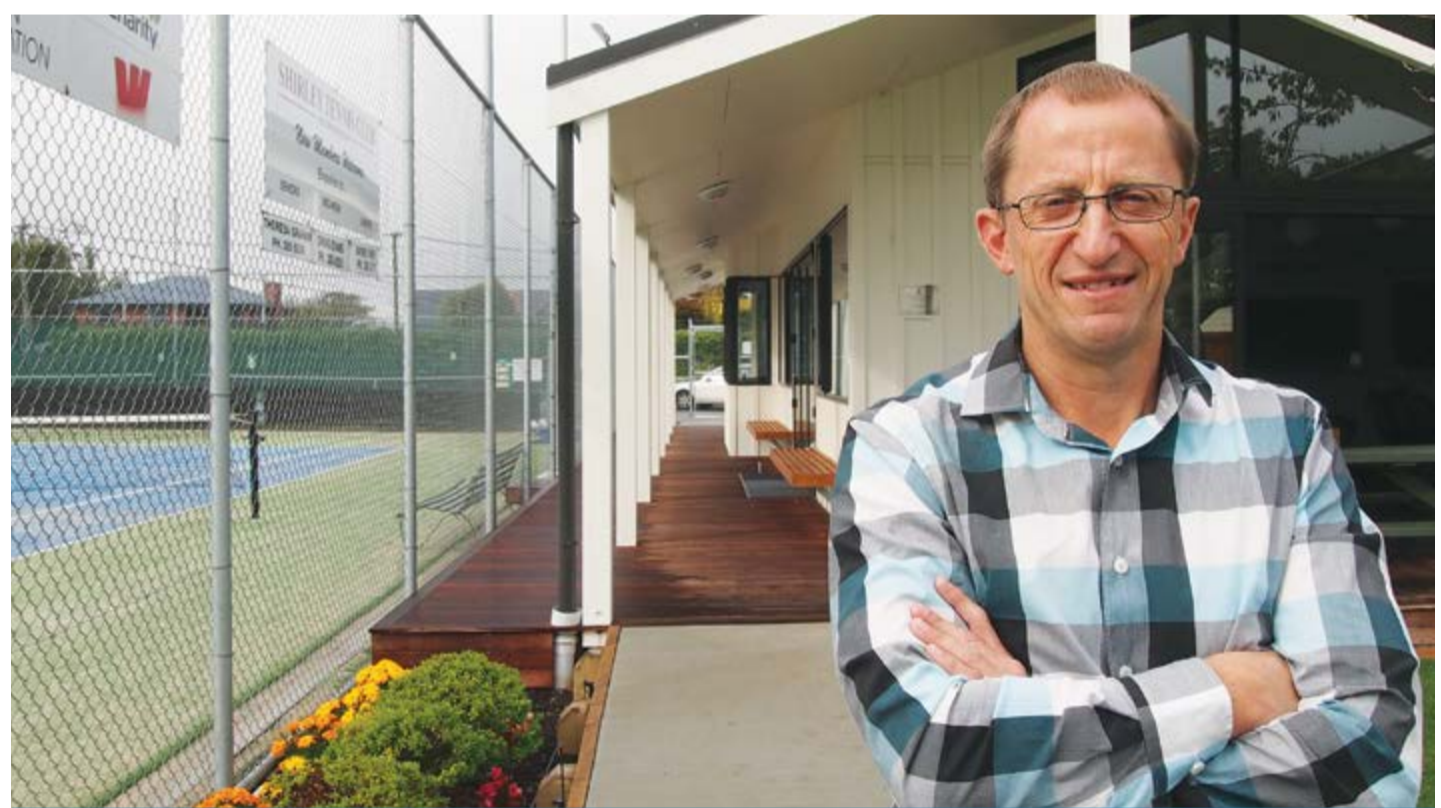
Wayne Turner at Shirley Tennis Club's new lightweight pavilion built on ribraft foundations.
