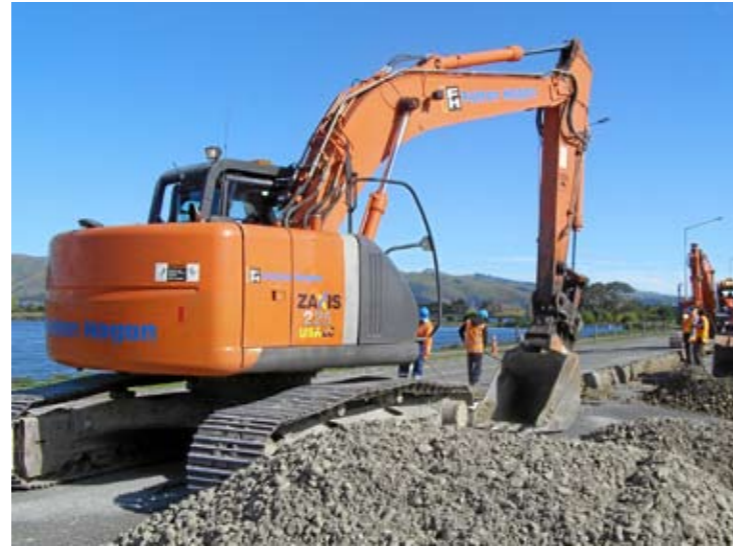
Trenches are dug out for underground infrastructure work on Anzac Drive.
