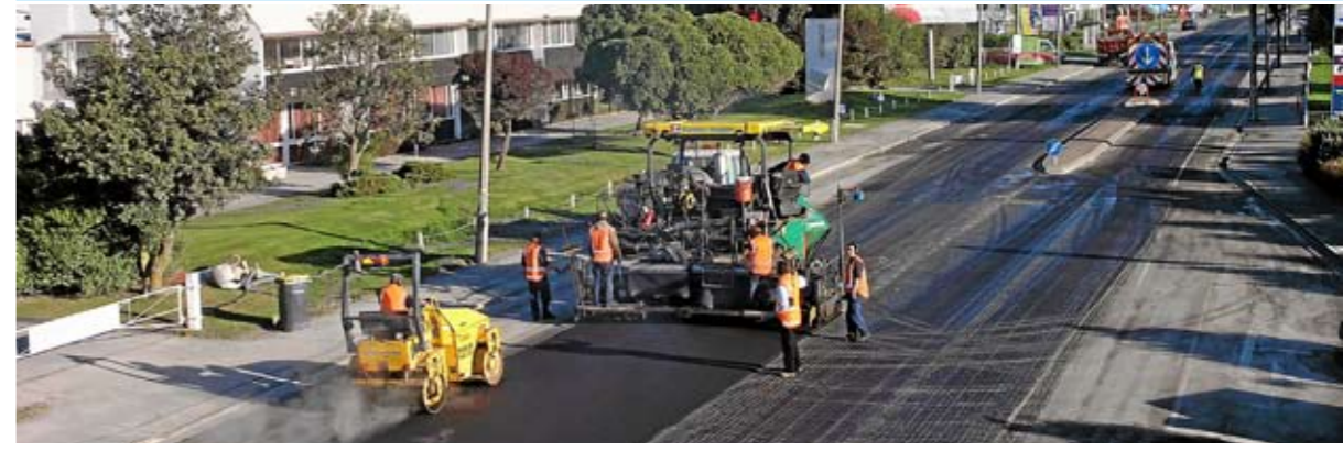
Crews lay down seal following road works on Ferry Road.
