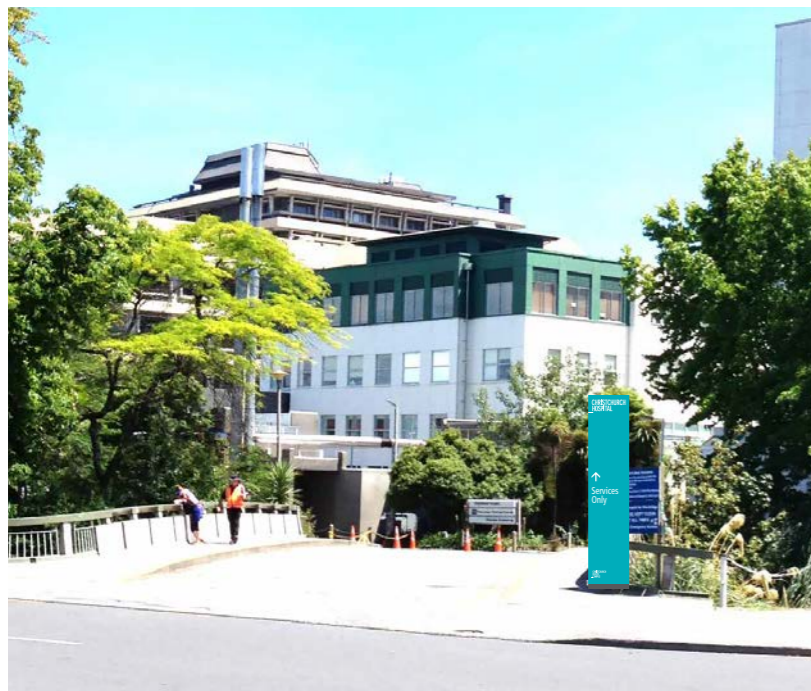
At intersection Oxford Terrace and Antigua Street. Service Entry.
