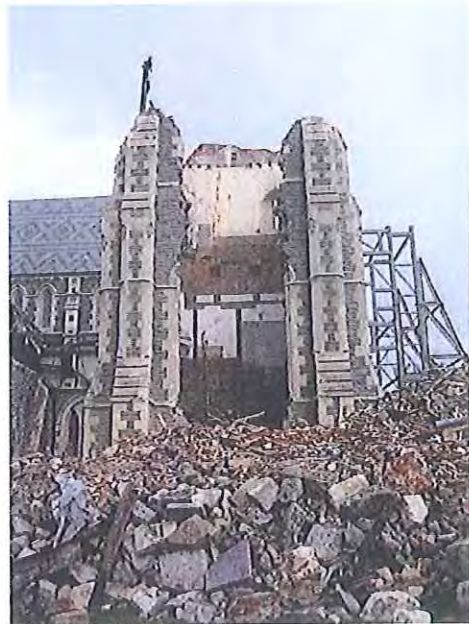
Figure 3 Damage Observed to the Cathedral Tower
