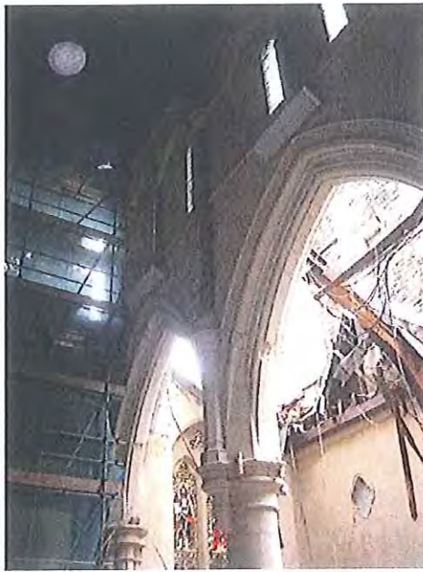
Figure 7 Damage Observed to the Nave
