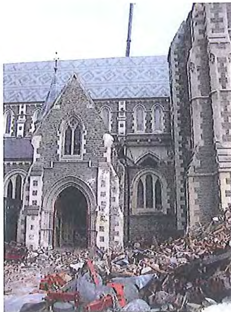
Figure 4 Damage Observed to the North Isle
