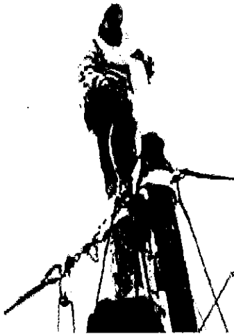
A sailor sending topmasts aloft. Standing on lower masthead, the sailor sets shrouds in place and assures that the topmast and rigging leads fair. Crew on deck mans the capstans to provide power to lift topmast. Note safety harness.
