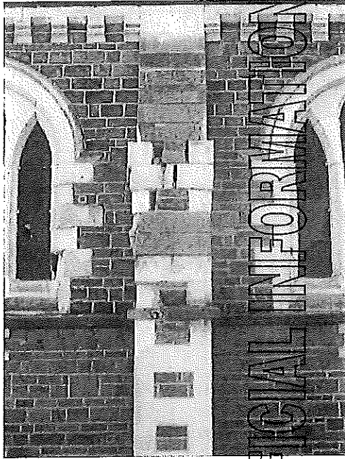
Figure 4 Damage Observed to the South Wall
