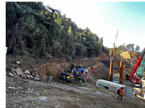
Taparahi Bridge works SH25A, Coromandel
