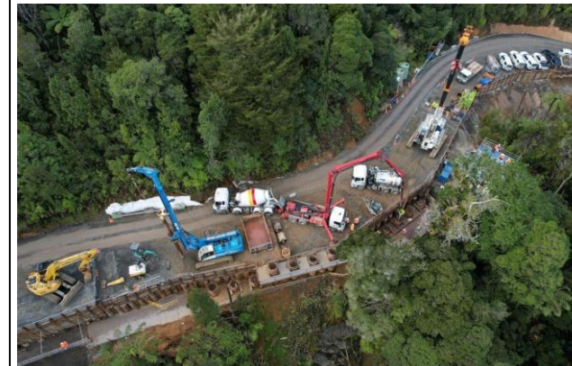
Mangamuka Gorge works SH1, Northland
